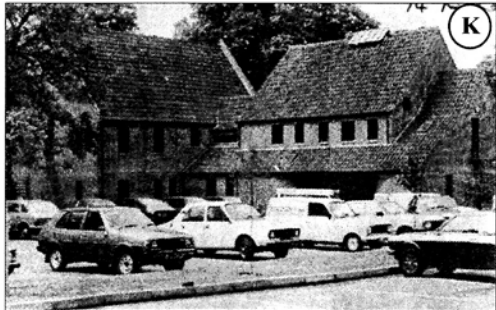
Breckland council's offices at Dereham (Guildhall). (taken from Dereham & Fakenham Times 14.10.1983).
