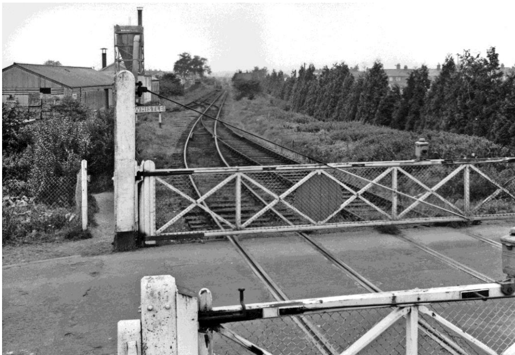
Looking west from Dereham West signalbox steps with the closed line to King's Lynn on 4 October 1969. All of the signalling had been removed by this time, but the level crossing remained in use in order to access Jentique's sidings and as a headshunt for the coal sidings. The EA station would have been where the bushes and whistle board are on the left. In the distance the Southend/Baxter Row level crossing can just be made out. The station site is now the car park of the Lynn Hill Guest House.
