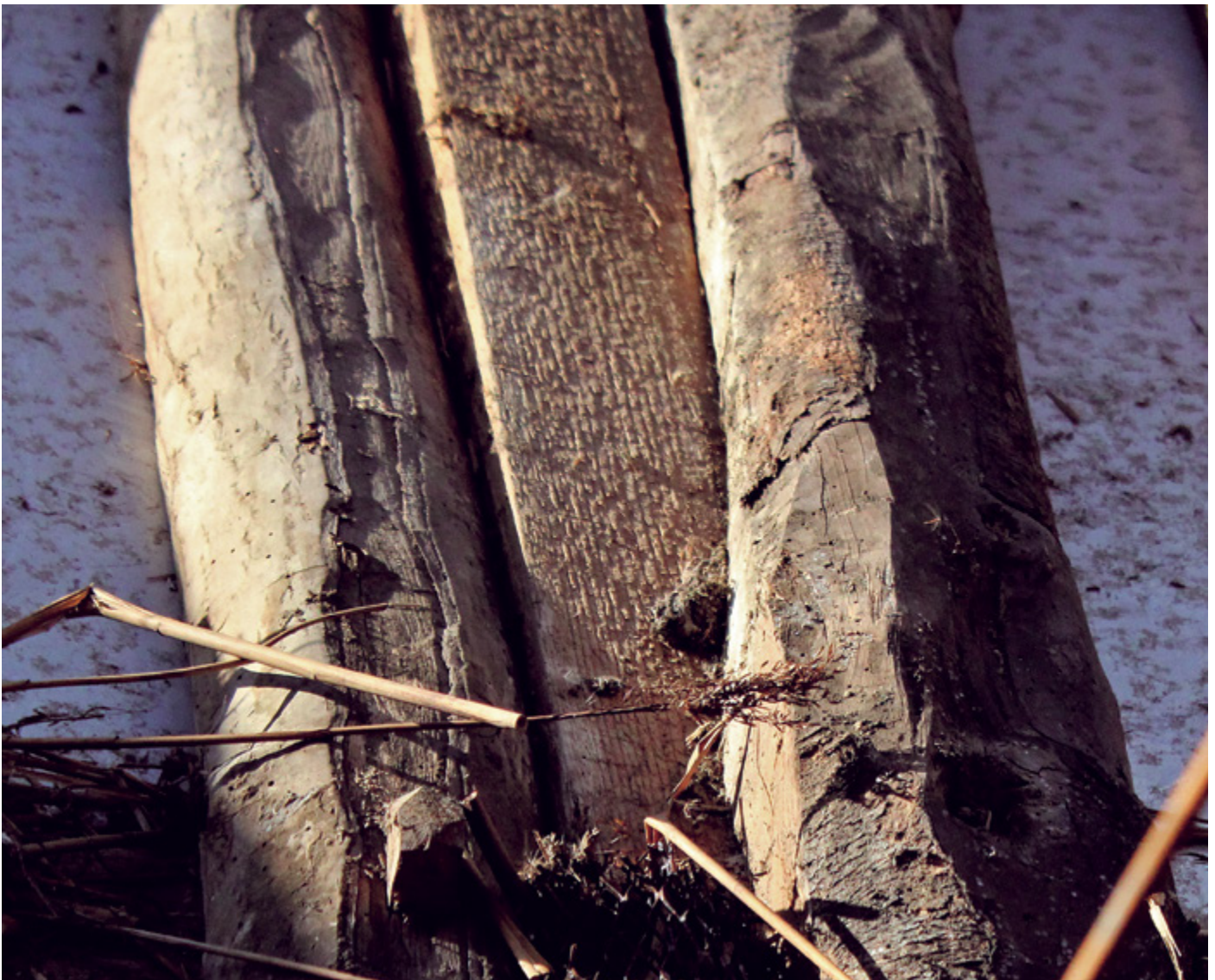
The photograph below shows three timbers from the East face of the roof. The central timber is a modern replacement roof timber cut with a machine saw. The timber on the left and right have both been hand shaped with an adz.
