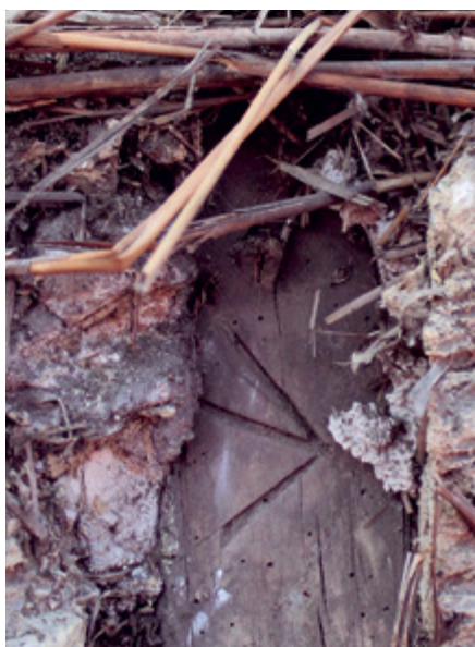
Above - The carpenter's arrow-like mark used as a symbol for the number 9. Two halves of a timber joint would be marked with the same symbol in the workshop, so they could be match up in pairs again on site.
