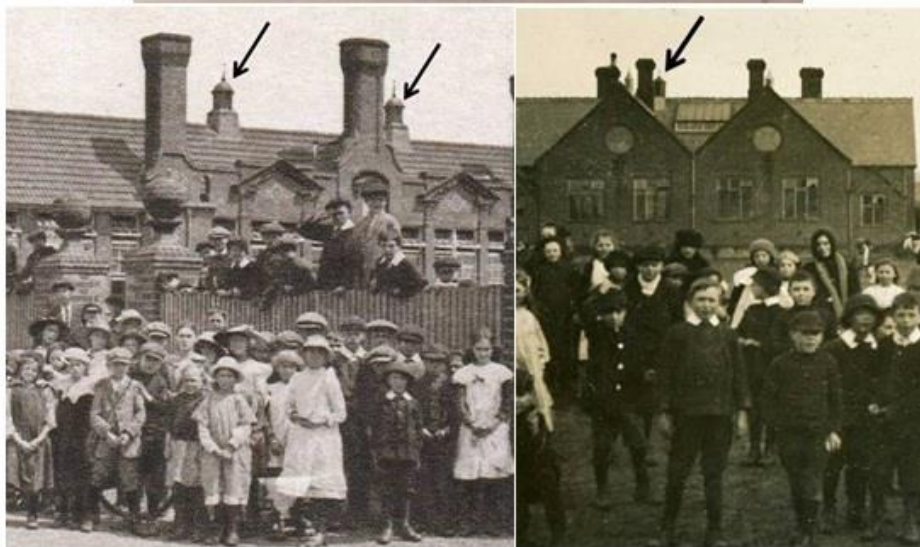
Toftwood, Crown Road, and Shipdham schools, and their ventilation cowls.
