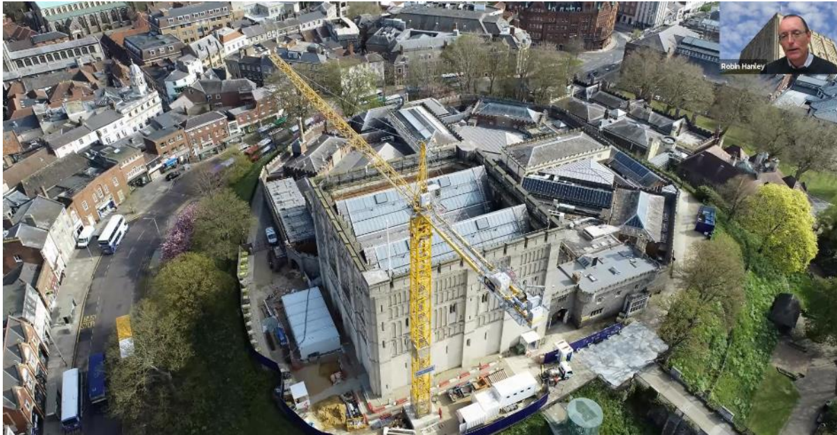
drone photo Perspective Media Ltd for Falcon Tower Crane Services Ltd
