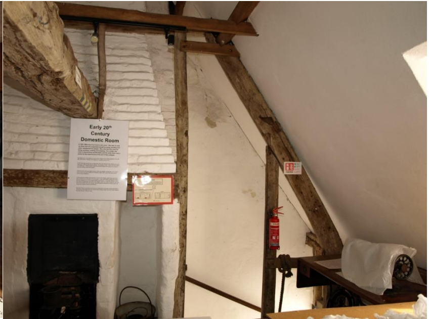
Top of truncated principal truss in north cottage
