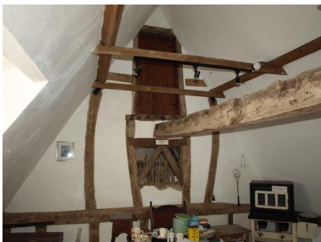
Queen post truss in the north cottage
