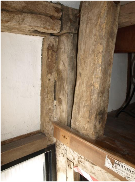
Bottom of principal truncated truss in north cottage
