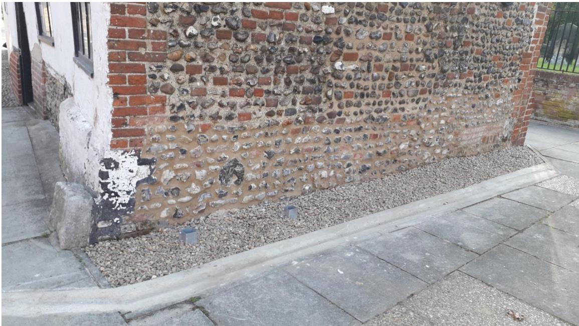
Improvements to deal with damp in the north wall
